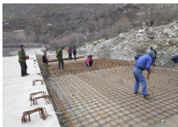
Figure 8. Typical At-Grade Open-Tray Crossing Under Construction
