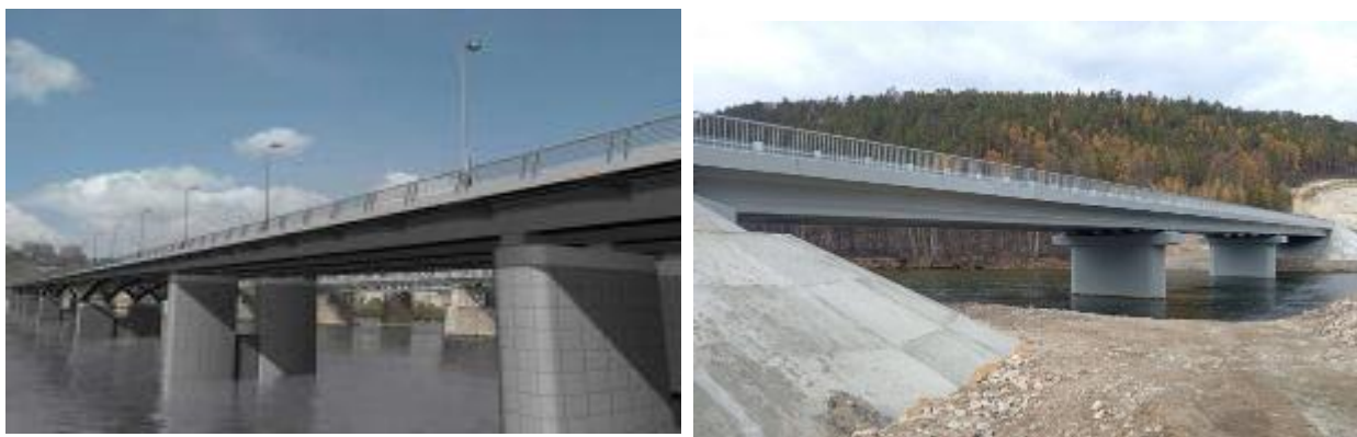
Figure 5. Bridges Similar to the New Bridges
