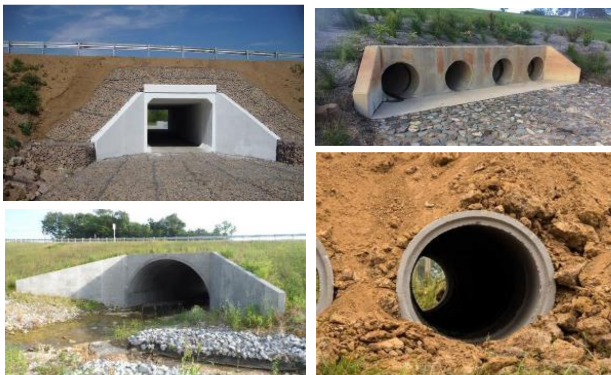
Figure 9. Typical Pipe and Box Culverts
