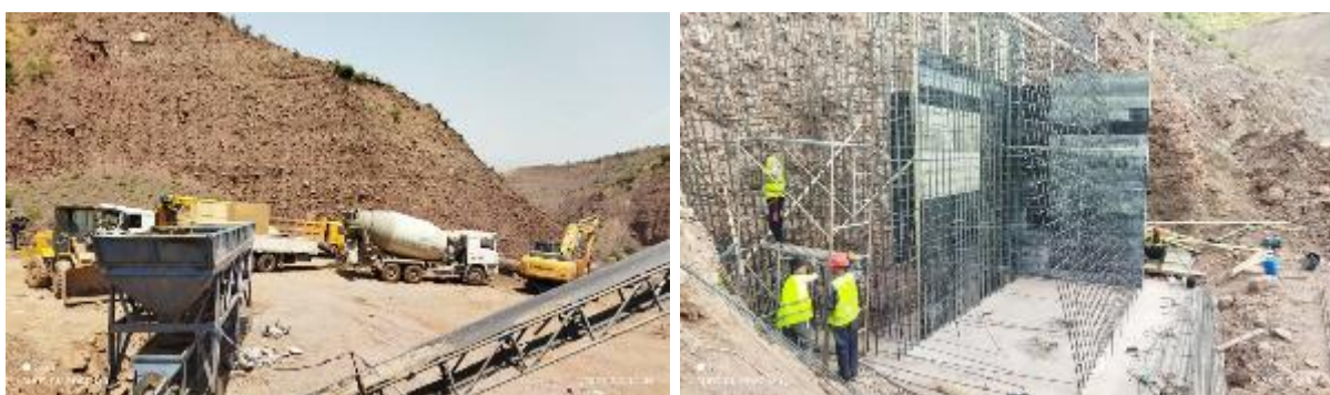
Figure 11. Ongoing Construction Considered Typical of Future Construction (Bridge Pier at right)
